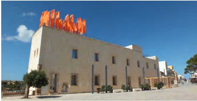
Lampedusa, building of the temporary exhibition Toward the museum of trust and dialogue for the Mediterranean . © Paola Boccalatte, 2016
