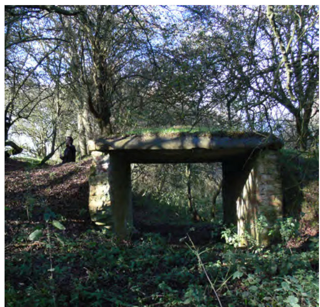
The remains of the earthwork blast walls protecting one of the filled shell magazines. The tunnel structure on the right is a portal through which the narrow gauge tramlines would have transported trolleys loaded with shells, ready for the trains. Photo: Dale Johnston ©Banbury Museum
