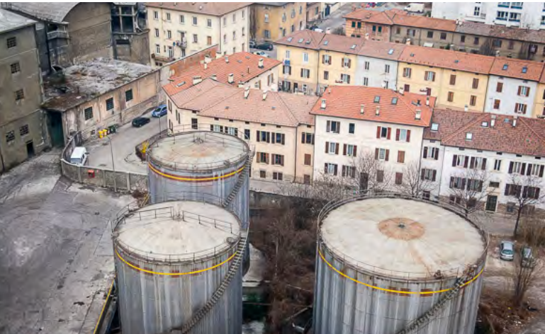
View from the cable car: tanks and workers' houses. Photo: Pierluigi Cattani Faggion
