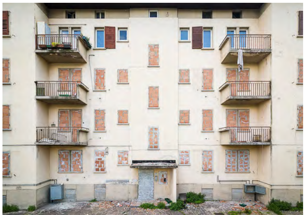
A workers' house next to the factory. Photo: Pierluigi Cattani Faggion
