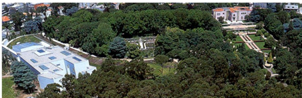
Figure 1 - Serralves Villa overview – Casa de Serralves on the right and the SMCA on the left
